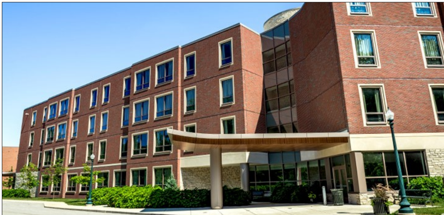
Rose-Hulman's Lakeside Residence Hall to have no student residence on the first floor next year
