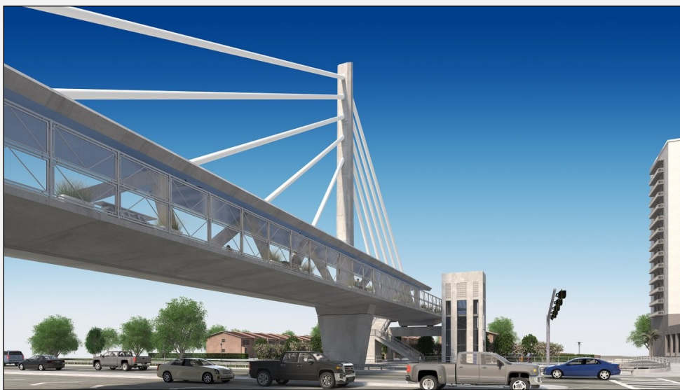
A 3-D rendering of the final bridge. Note the large cables meant to relieve the tension on the underside of the bridge.
