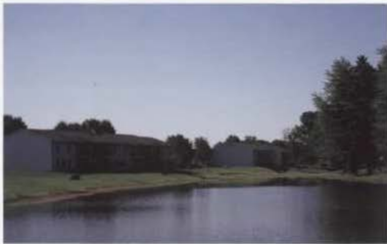
(Left) The Heritage Trail Apartments are another option for those looking to leave Residence Hall life.
