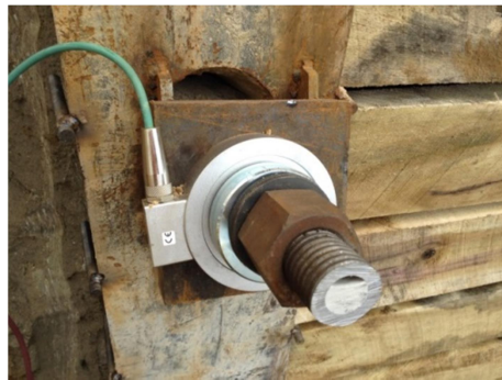
Figure 5.3: Load Cell Installed at a Tieback
