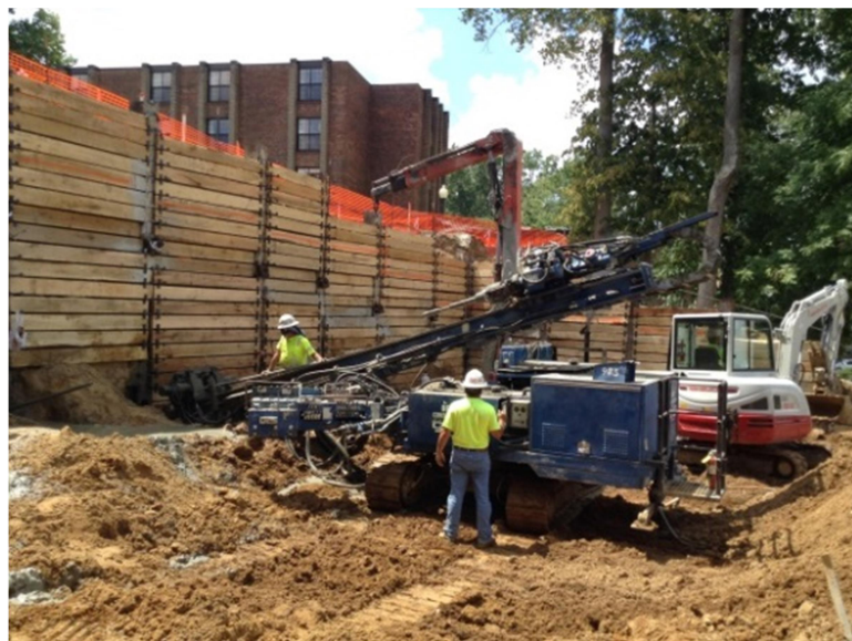
Figure 2.4: Installation of Tiebacks (08/11/2016)
