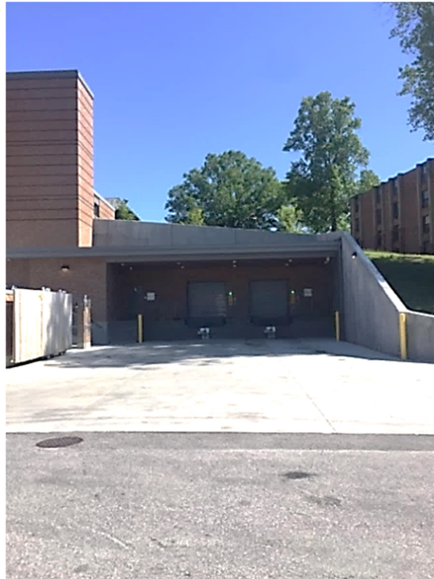
Figure 2.6: Wall After Construction (06/05/2018)
