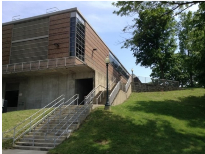
Figure 2.2: Northwest Corner of the MU Before Construction (05/25/2016)
