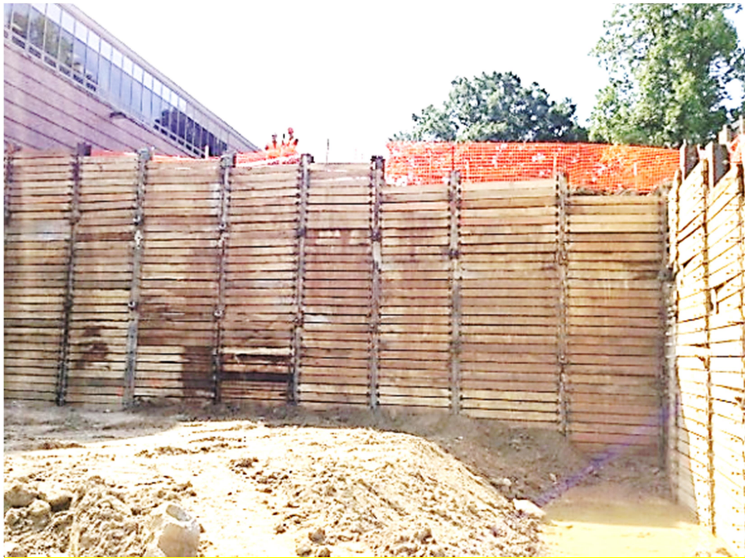
Figure 2.5: Completed Wall before Concrete Facing (08/29/2016)
