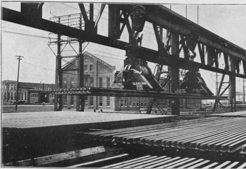
Rail Handling Magnets at the Gary Works of the Illinois Steel Co. Total Weight of Load, 23,000 Pounds.
