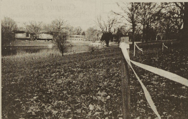
The construction company has already set up stakes and construction material on the new residence hall. Foundation work is set to begin within the next few weeks.
