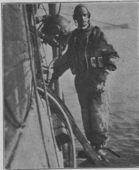
NEARLY READY TO GO DOWN (Hyperion Pipe Job, So. Calif. Coast)
