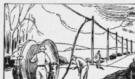
CONSTRUCTING THE LINE
