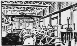
MAKING THE CABLE
