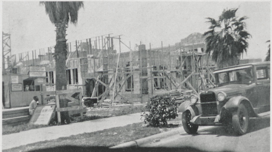
View of building showing formwork for reinforced concrete.
