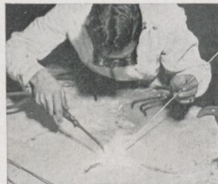
WELDING ALUMINUM—an architectural plaque, modern in design, is repaired by a modern method.
