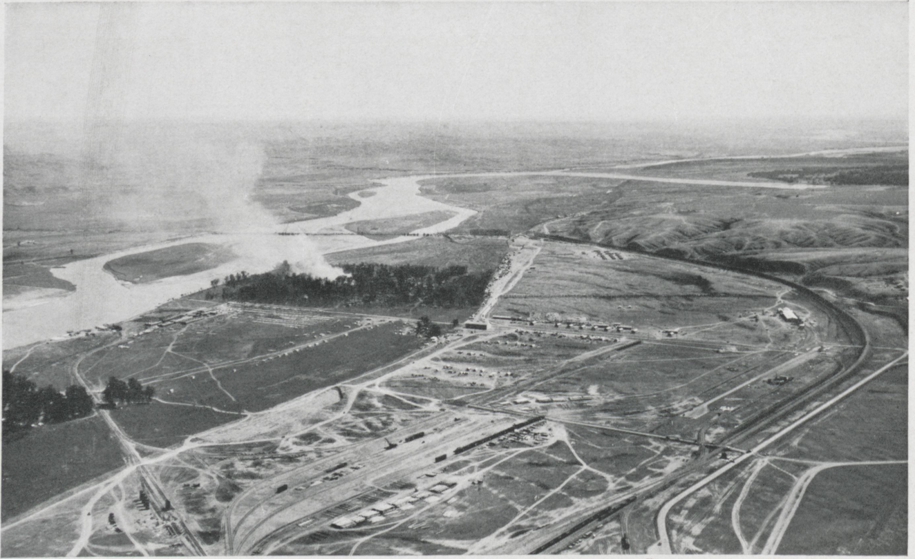
View of the Fort Peck Dam Site.
