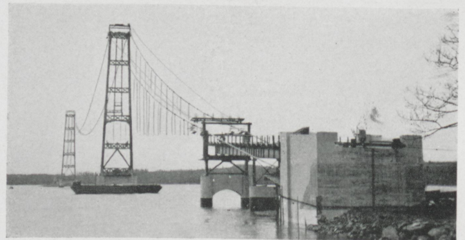
A partially completed Suspension Bridge.
