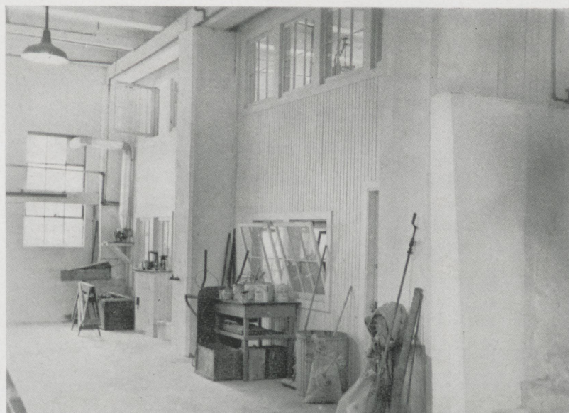
PARTIALLY COMPLETED HYDRAULICS LABORATORY
