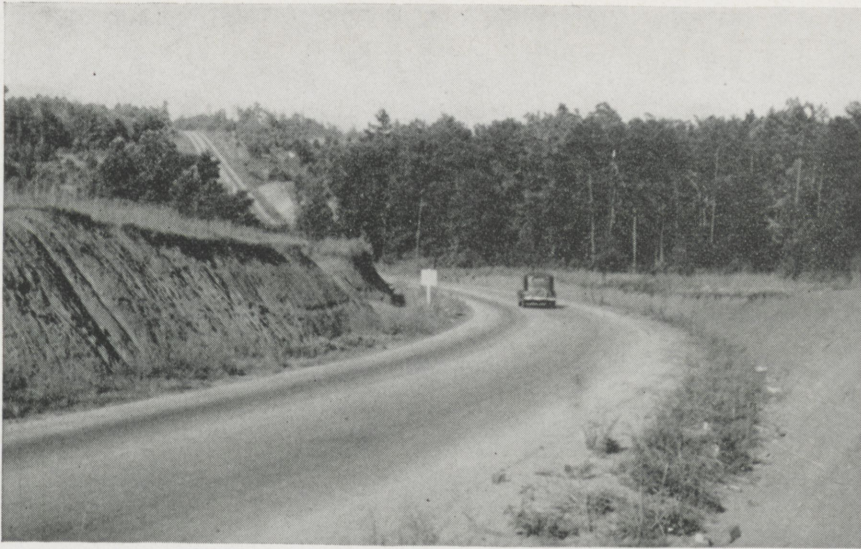
Two Lane Highway before improvement.
