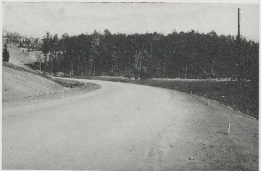
Same Highway after faults have been corrected.
