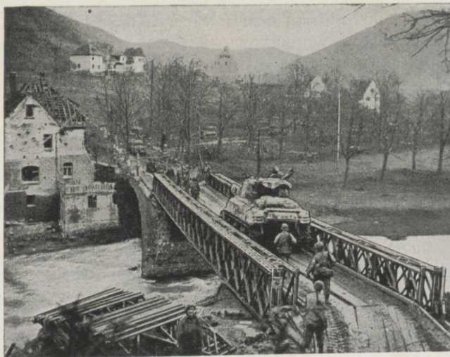
110-foot triple truss single-story fixed Bailey over the Roer River at Heimbach, Germany.
