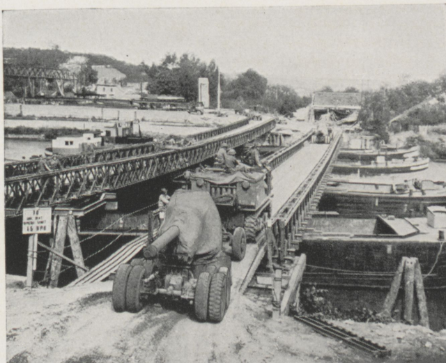
Two-lane Bailey on barges over Seine River
