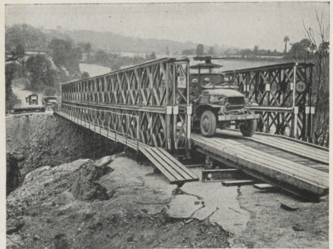
110-foot triple-truss double-story fixed Bailey over Vire River near Vire, France.
