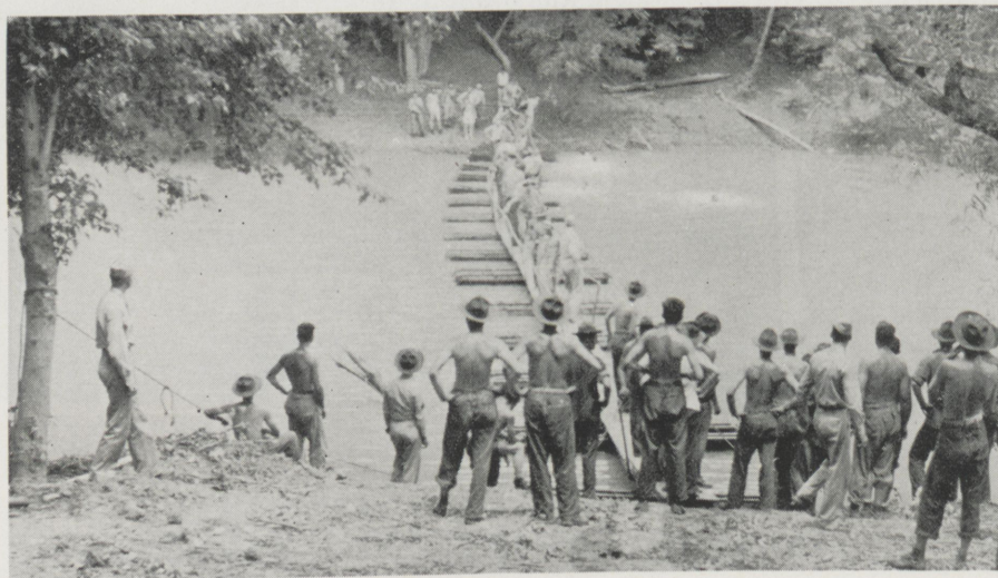
R.O.T.C. Engineers build footbridge at summer camp in 1940. Post-war summer camps are scheduled to begin next year.
