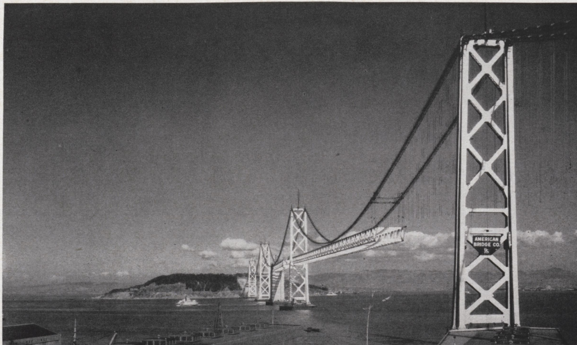
San Francisco—Oakland Bay Bridge During Construction
