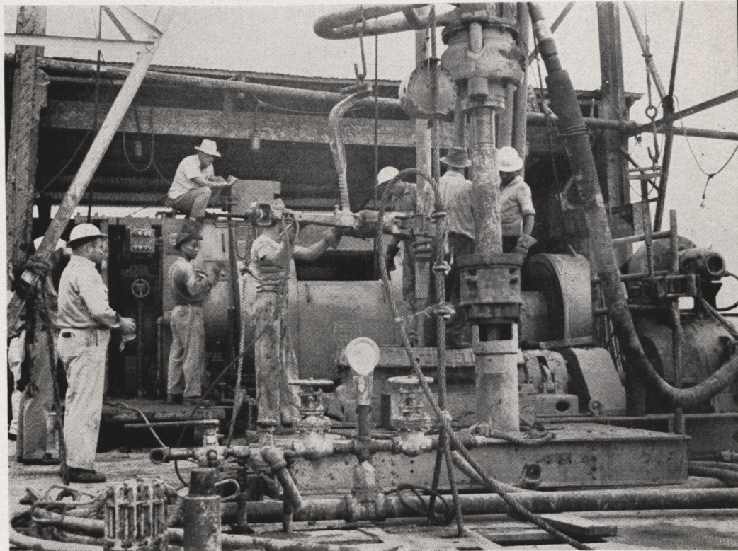
Drilling Crew At Work
