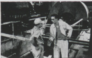
Philo, Ohio — MECHANICAL ENGINEER Alan G. Lloyd helps supervise installation of world's first super-critical pressure generating unit.
