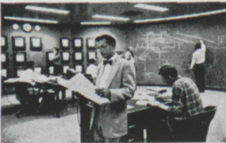
Canton, Ohio—SYSTEM OPERATION ENGINEER Richard P. Blaes helps to coordinate load scheduling and the exchange of power with other electric utilities.
