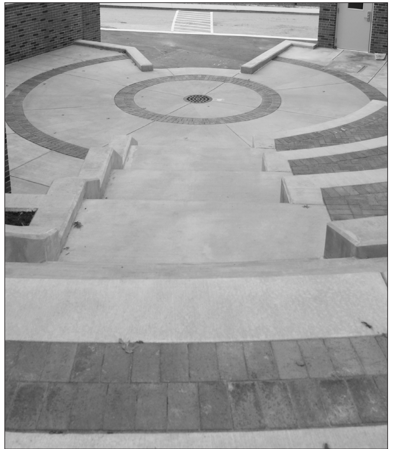
Just before quarter break, construction wrapped up in the quad, revealing a set of concrete steps between Crapo Hall and the library, featuring a new entrance to the second floor of Crapo.
